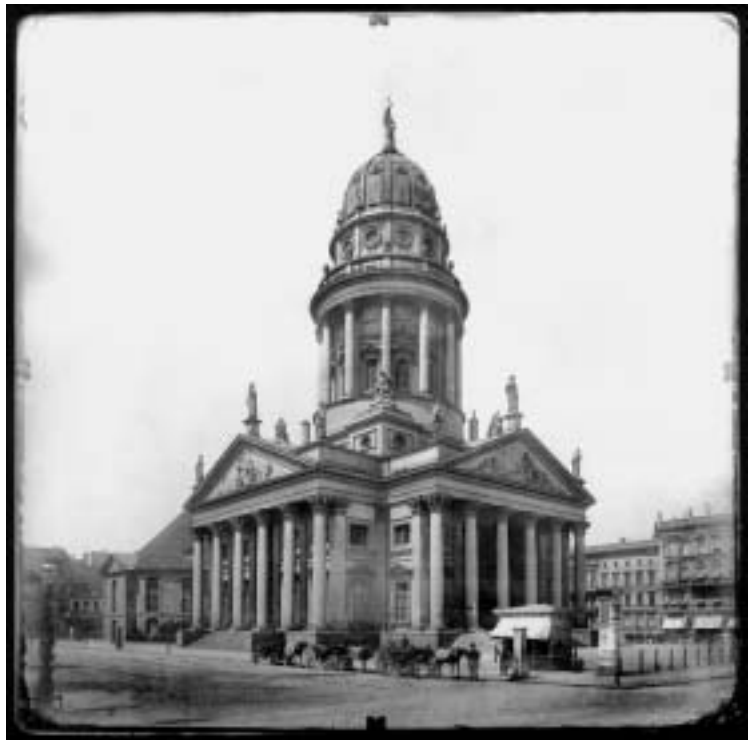
Fig. 4: The French Cathedral in Berlin. One of Meydenbauers experimental photographs from 1882 (40 x 40 cm). 100 years later, between 1977 and 1982, the image was used for the reconstruction of the church which was severely damaged during World War II.
